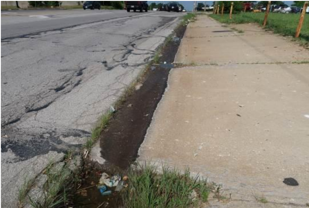
Deteriorating Roadbed, Gutters, Curbs, & Sidewalks Along E 63 rd Street
