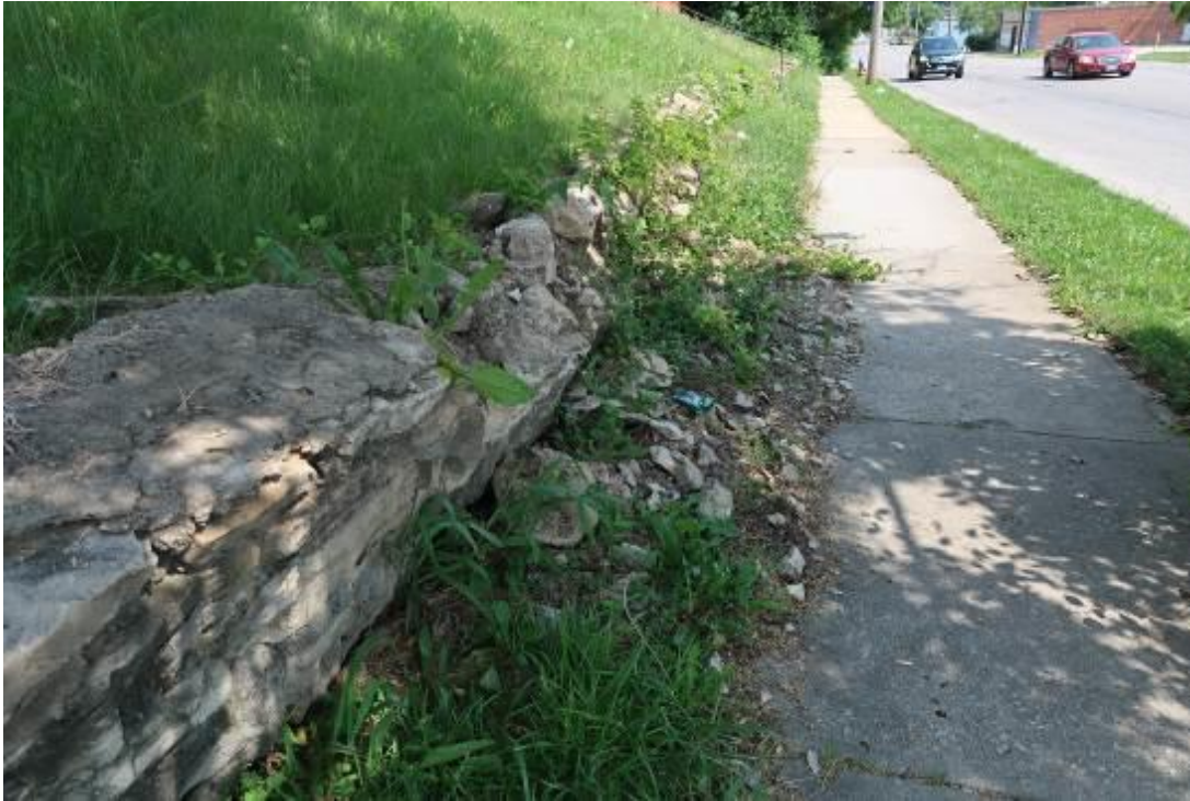
Collapsing Retaining Wall Along Pedestrian Sidewalk On Prospect Avenue
