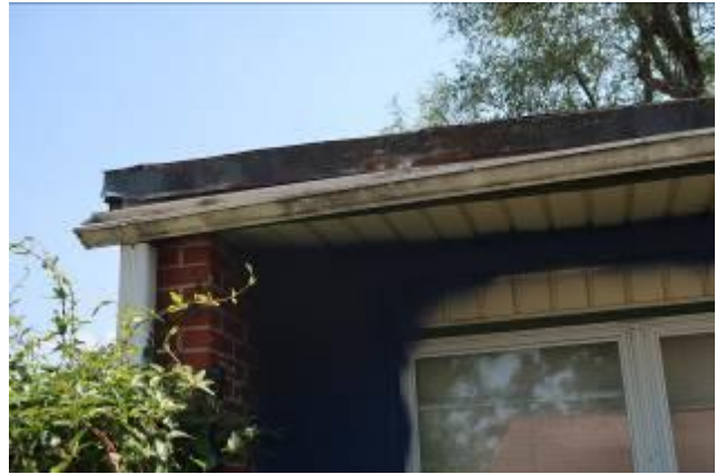
Guttering Damage
