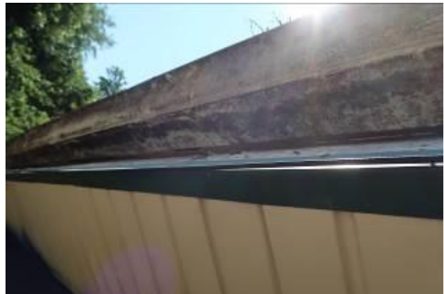
Guttering Damage
