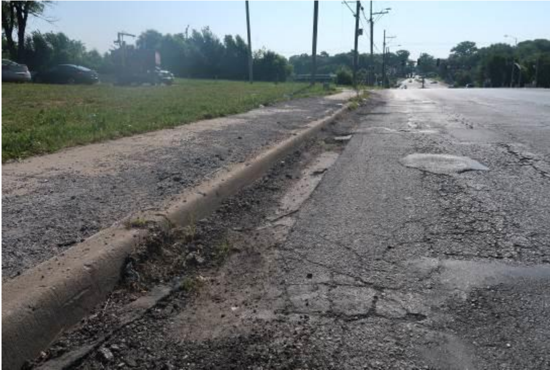
Deteriorating Roadbed, Gutters, Curbs, & Sidewalks Along The North Side Of E 63 rd Street
