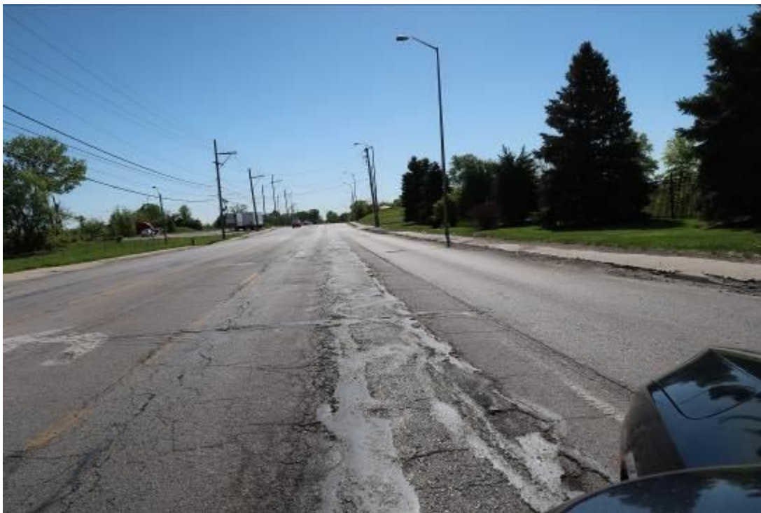
Deteriorating Roadbed In The Center Turn Lane Of E 63 rd Street
