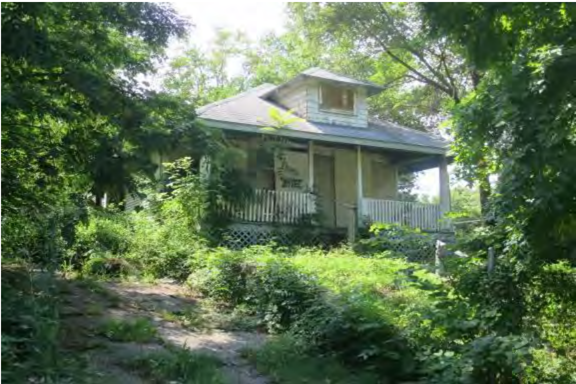
Dangerous Building Citation (SWC Agnes & 49 th Street) – South Of Study Area
