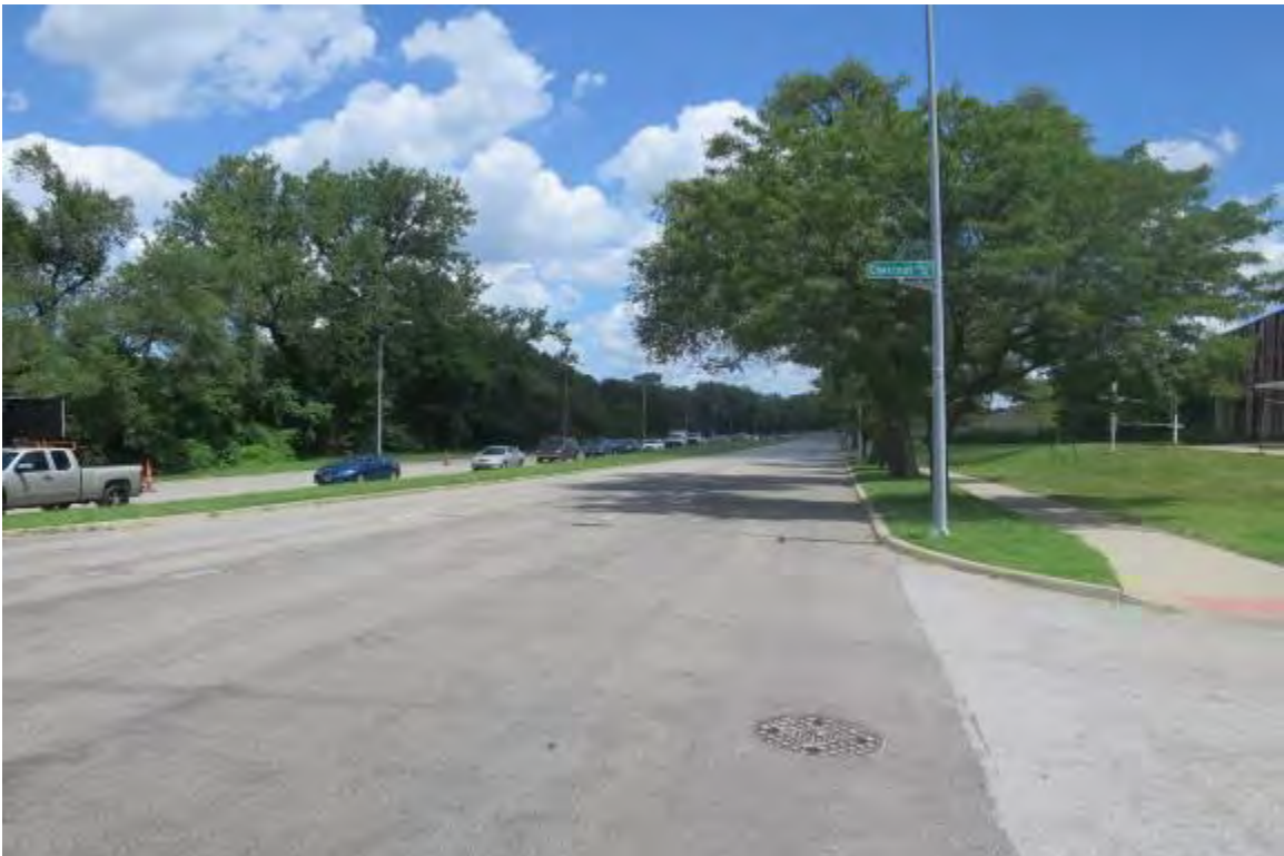
A View East On Swope Parkway From Chestnut Avenue
