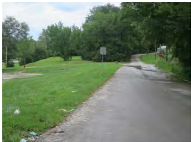
Lack Of Sidewalks E 49th Street
