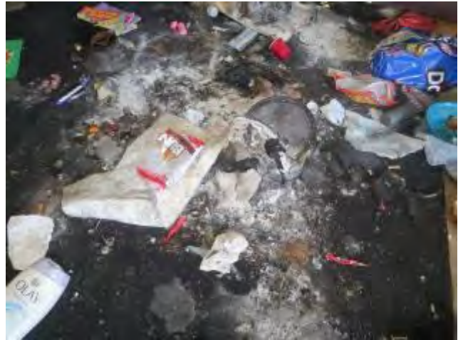
Interior Fire At 2801 Swope Parkway
