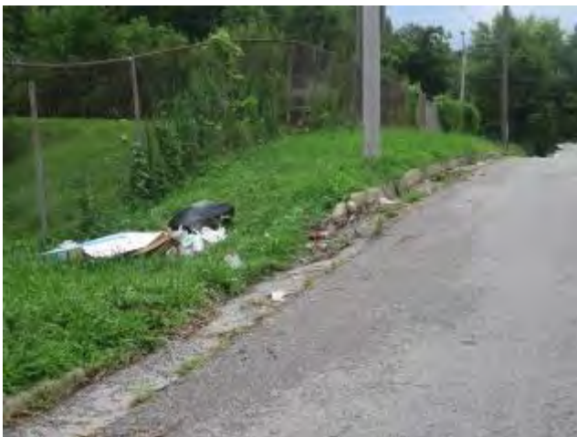
Lack Of Sidewalks Chestnut Avenue
