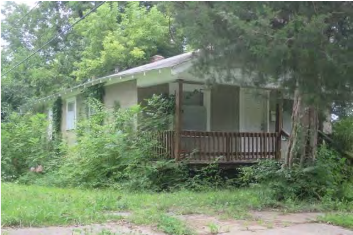
Vacant Boarded-Up House On North Side Of E 49 th Street (2914) Adjoining The Study Area
