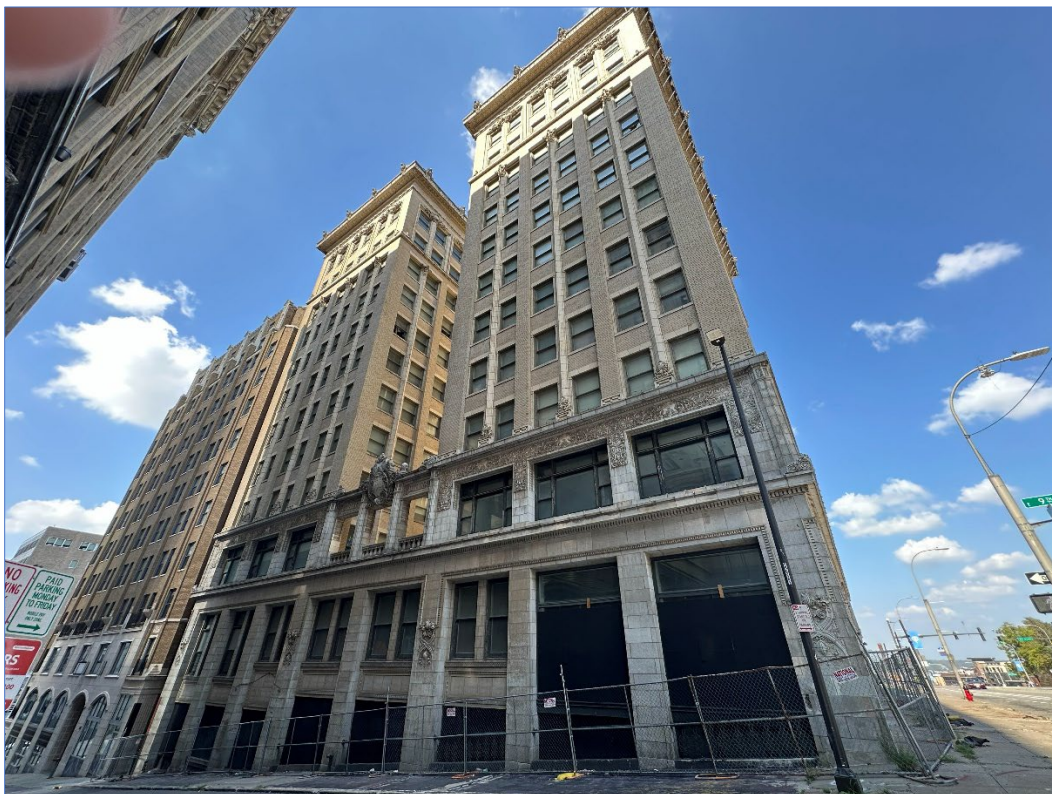
818 Grand Blvd (Scarritt Building) – looking northwest
