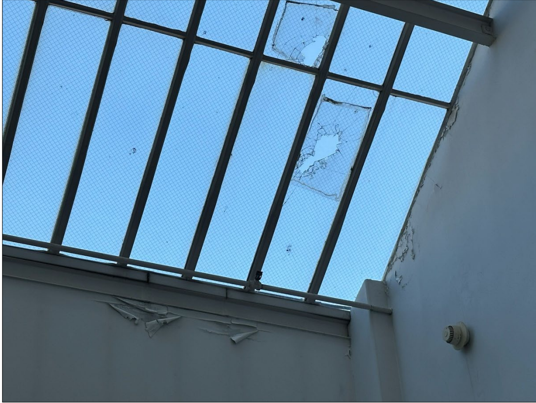
819 Walnut St – looking north – damaged glass panels in roof; failure of finishes
