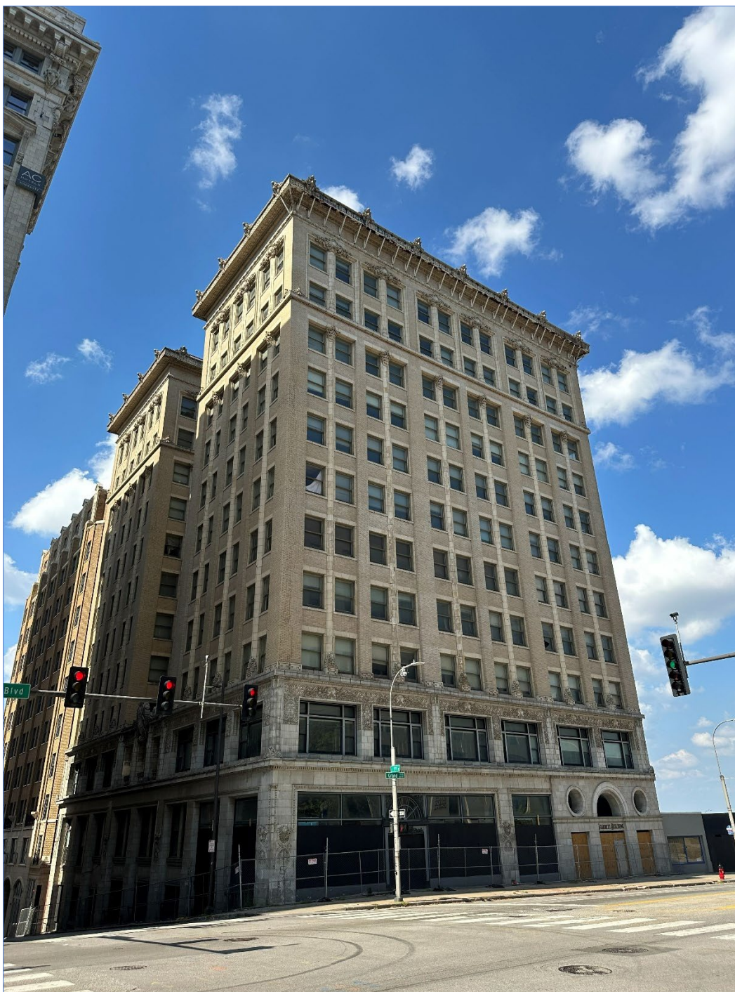
818 Grand Blvd (Scarritt Building) – looking northwest
