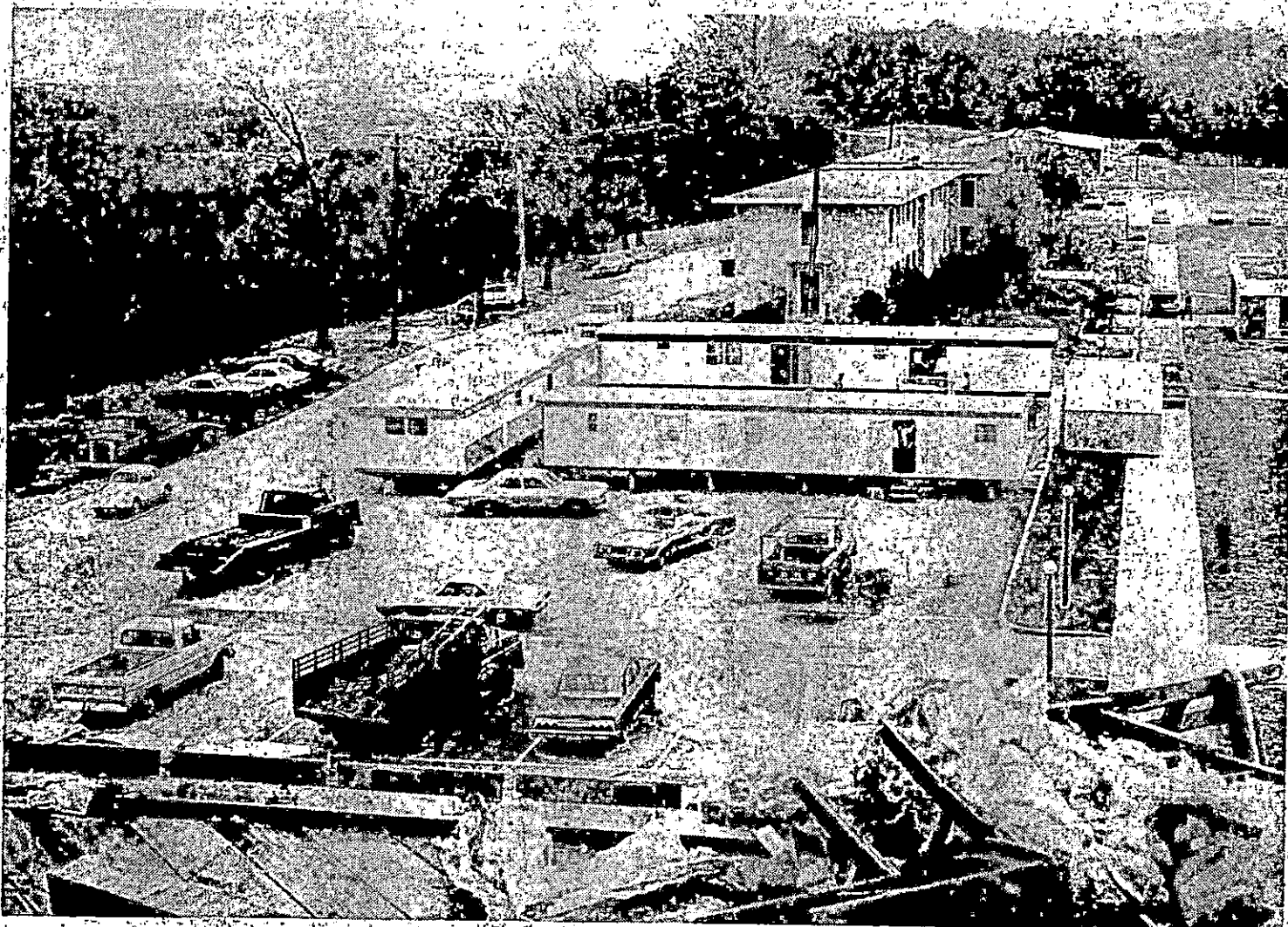
TEMPORARY OFFICES —Arkansas College officials wasted no time in setting up administrative offices in rented trailers in a campus parking lot after a tornado inflicted heavy damage to several buildings April 19. The picture was taken from a ripped-out portion of the administration building.
