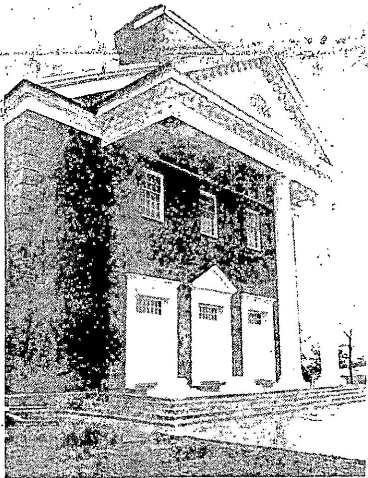
Arkansas College Chapel heavily damaged
