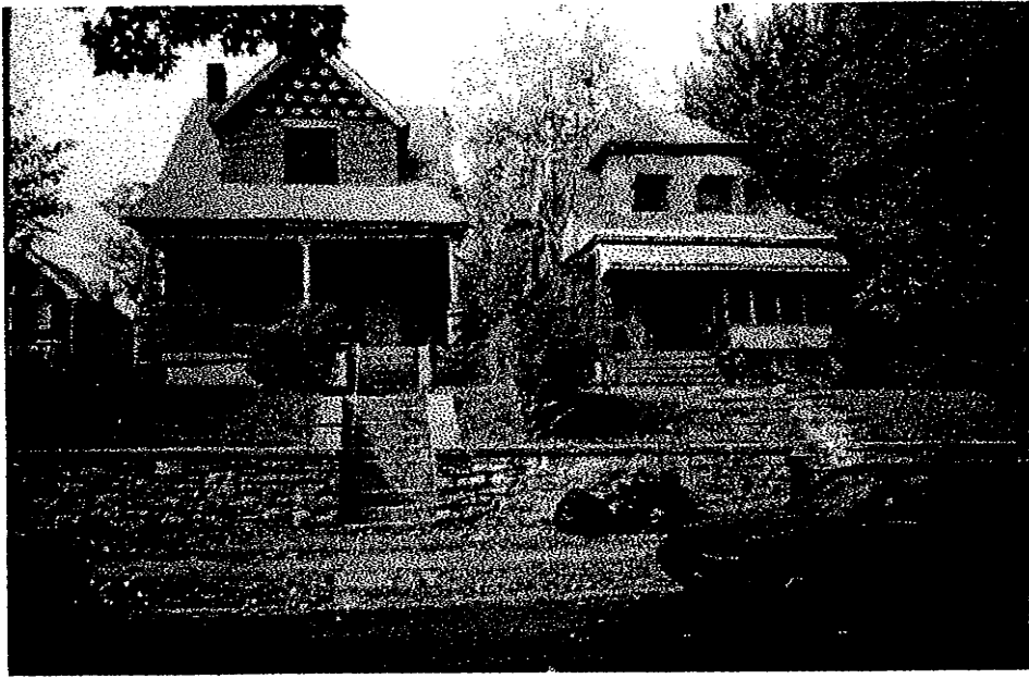
2318 & 2320 Park. 2320 is vacant. 2318 is occupied. These are the only two homes along the West side of Park between 23 rd & 24 th Streets. Purchase/demolition is recommended for both structures.
