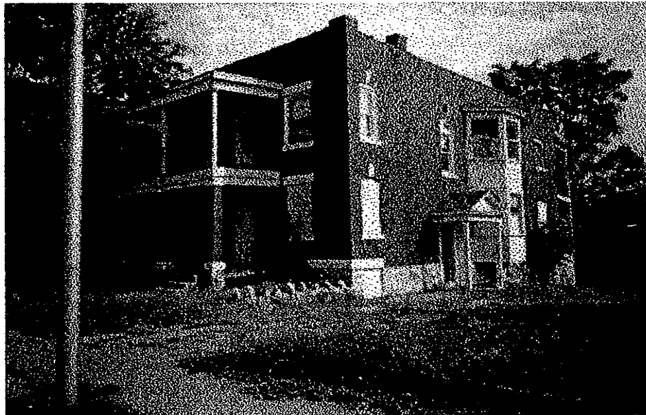
2307 Brooklyn – Vacant, probable beyond repair.
