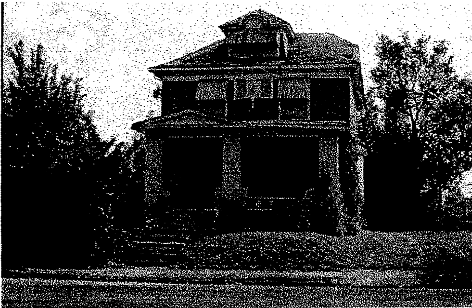
2329 Brooklyn – Vacant, probable beyond repair.
