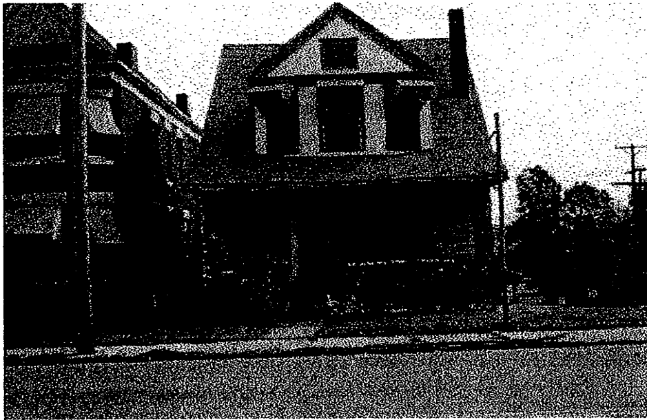
2223 Brooklyn – Vacant, possible candidate for purchase-rehab, but may be beyond repair.
