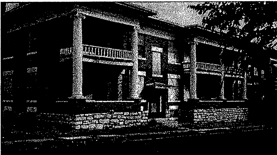
2202 E 24 th – Vacant multi-family complex. Feasibility of rehab is unknown, but doubtful.
