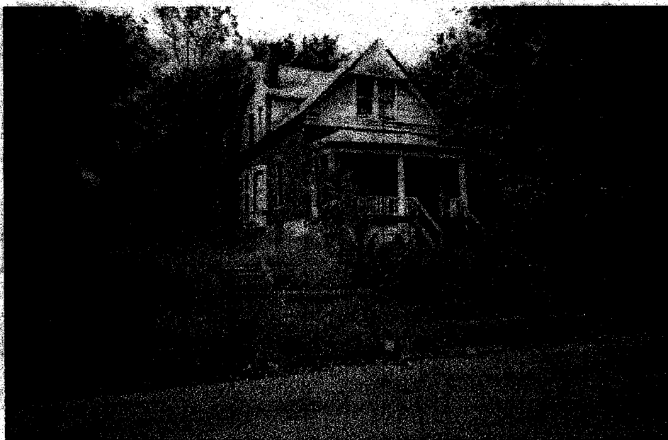
2118 Park – Vacant structure. Possible purchase/rehab.
