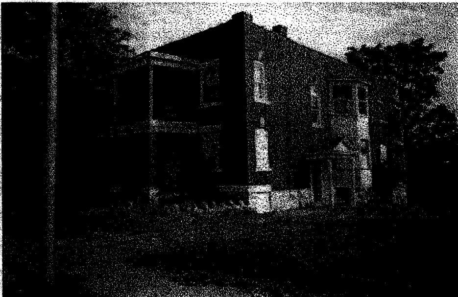
2307 Brooklyn – Vacant, probable beyond repair.
